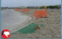
Piles of sediment are inappropriately placed on top of ECBs in the process of digging for utility/water lines.
