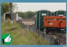
Portable toilets are placed behind BMPs and away from the street or drainage ways should a spill or leak occur.
