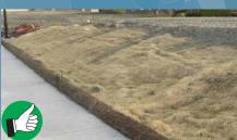
Organic filter tubes are used with other BMPs to protect an area that may prevent the embedment of other controls.
