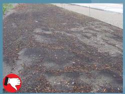
Mulch was applied in an area of concentrated flow and is washing away. Mulch should be applied evenly and uniformly and at an appropriate thickness.
