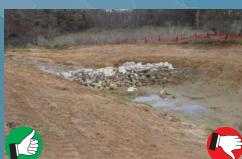
Check dam is effectively removing sediment; however, debris should be removed from the dam. Outer edges at channel sides must be higher than the center overflow point.
