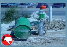
Chemical storage container is inappropriately discarded, and there is evidence of a spill. Chemicals should be properly stored and disposed of and spills cleaned up immediately.
