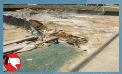
A washout area has been designated; however, the waste is being managed inappropriately. BMPs surrounding the washout area are damaged and the area is full and concrete should be removed and disposed of properly (recycle where possible). BMPs are absent to protect against offsite tracking and runoff.
