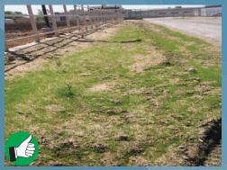
Mulch is applied to reduce sediment runoff. Mulch needs to be applied regularly in high traffic areas to maintain uniform thickness.
