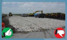
Good application of stabilized construction exit; however, offsite tracking is still occurring. Voids between stones may be filled with sediment. Fabric and rock should be extended to orange barrel to better transition to paved surface. Good use of barriers to ensure stabilized exit is used.
