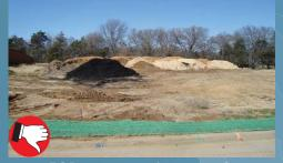
Inadequate ECB to protect this area of exposed soil; additional BMPs are needed. ECB is not trenched or anchored correctly as indicated by sediment at the curb. Spoil piles should also be better protected.
