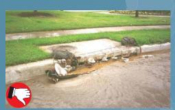
Poor management of filter fabric and wire mesh to protect the storm drain. Protection is bent and is not flush with the storm drain to properly pond runoff and filter out sediment. Maintenance is not being performed as needed.
