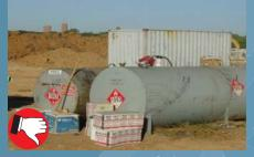
Inappropriate management of chemicals and other hazardous materials. Gas tanks need secondary containment that is 110 percent of the container. Other chemicals should be stored in an appropriate enclosure to minimize potential of stormwater contamination.
